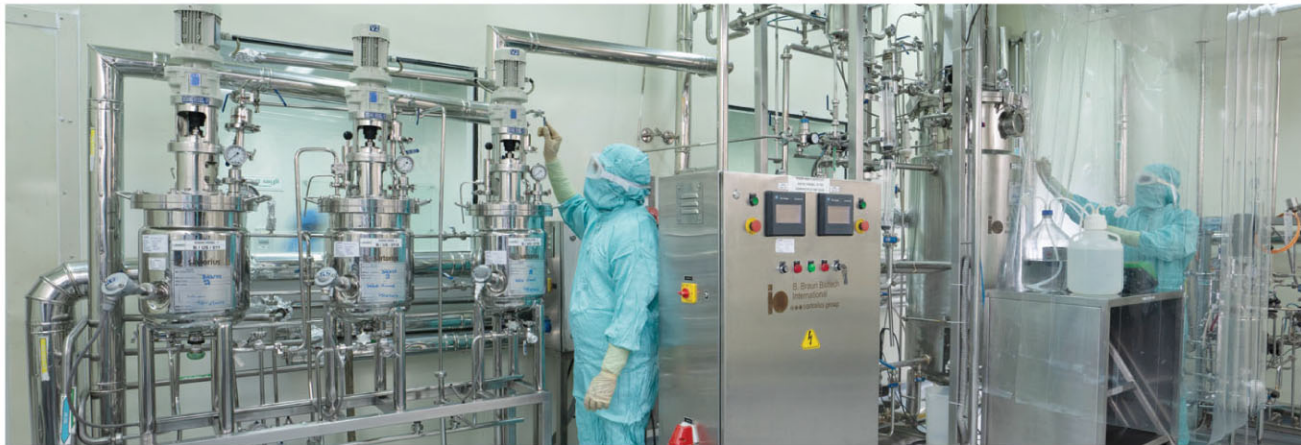
Fermentation and upstream process at GMP manufacturing plant at Puducherry.
